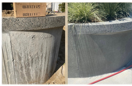
Before FirmeCrete® Wall Coating
