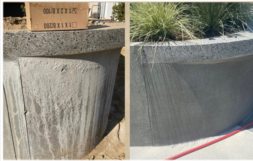
Before FirmeCrete® Wall Coating
